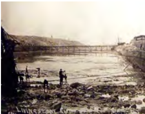
Construction of the Livingstone Channel in the Detroit River.
